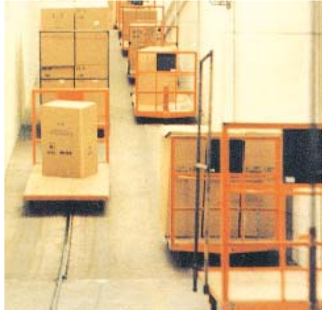
Towline conveyor system for carton transport
