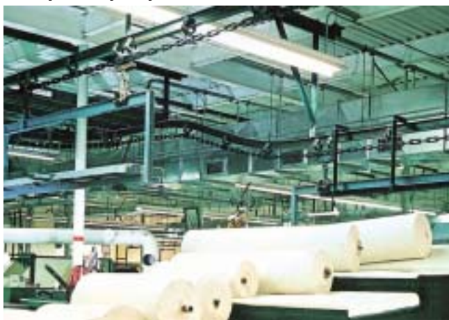
Trolley conveyor system
